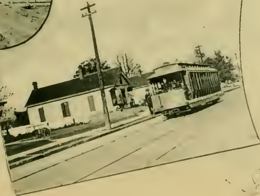
Electric Car on Eleventh Street.
